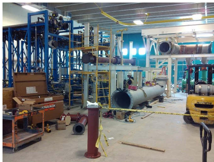
Pic. 2 – Piping connected to membrane system
