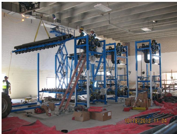
Pic. 1 – Moltz installing Pall membrane rack framing.
