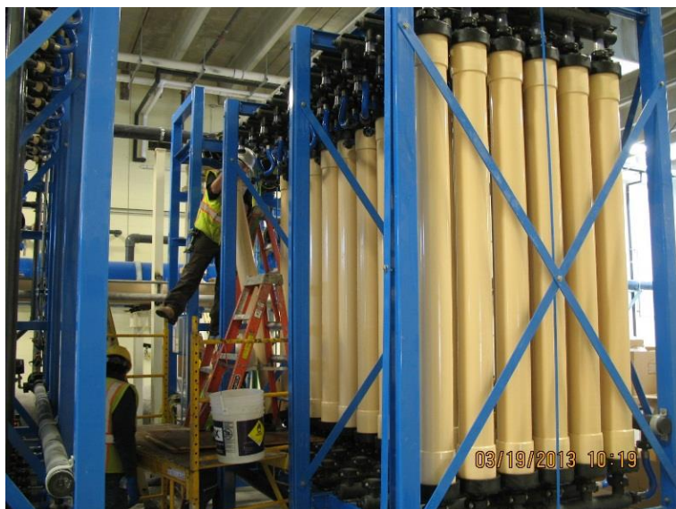
Pic. 1 – Moltz installing Pall membrane rack framing.
