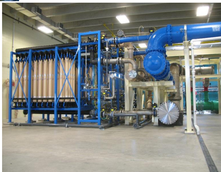
Pic. 4 – Final membrane system including electrical and SCADA controls completed and started up by Moltz Construction.
